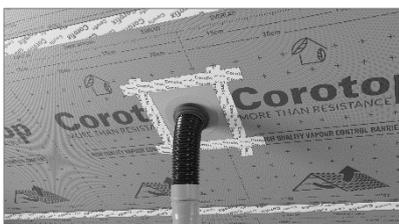
4. Seal all places where service lines pass through the vapour control layer (e.g. electrical cables, pipes, etc.) thoroughly with special adhesive or adhesive tape (e.g. Corotop FIX, Corotop BUTYL).
