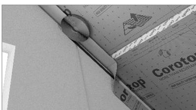
3. The places where vapour control layer connects to the wall should be sealed with special adhesive or butyl tape (e.g. Corotop BUTYL). It is recommended to use an additional hold down strip and to leave about 2 cm of excess foil (folds).
